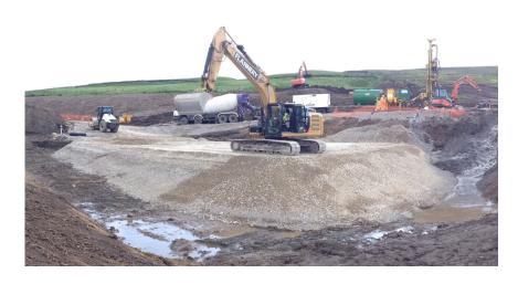
We were appointed to undertake the mine workings stabilisation and civil engineering infrastructure work for a single wind turbine development located near Burnley, Lancashire. The EWT DIRECTWIND 52/54—900kW (geared to 500kW) Wind Turbine generator has a hub height of 40m and is capable of generating between 1500—3000MWh/yr.
